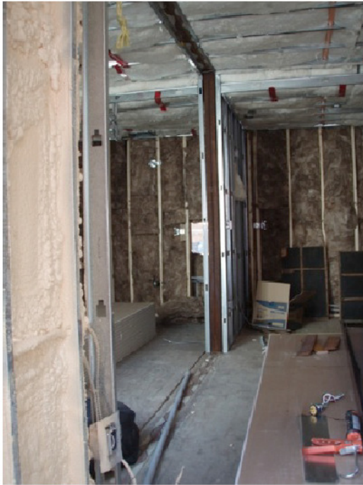
Fig. 5. Insulation to ceiling and walls. Source: JTW consulting [14].
