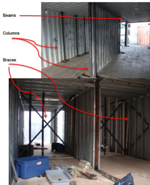
Fig. 4. Modifications in container, addition of reinforcement. Source: JTW consulting [4].
